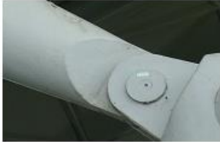
(a) Photograph of a clevis pin connection
