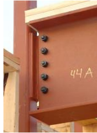
Web cleat connection Model as a pin
